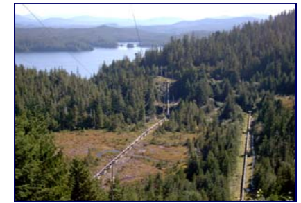
Beaver Falls Hydroelectric Project Environmental Support; AK
